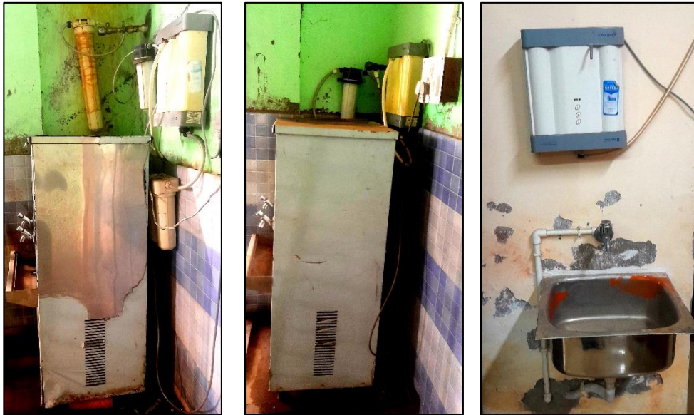
Figure : The filtered potable water units installed at Government General Degree College, Keshiary
